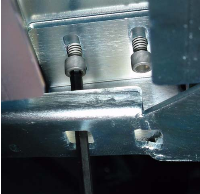
Figure 13. Attaching support rail from below
